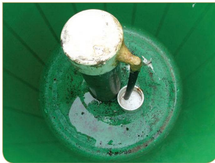
The construction of the bell
